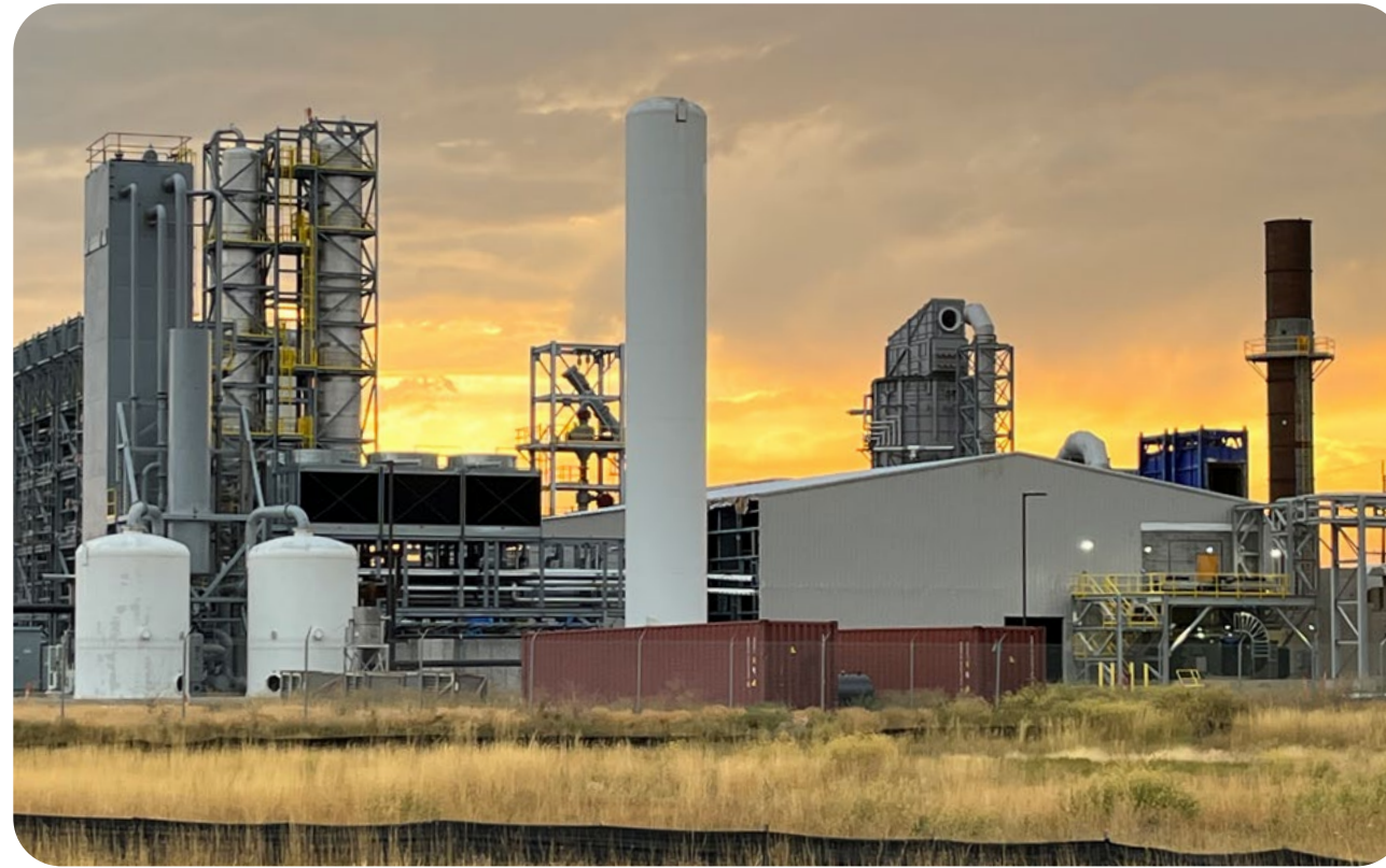
Lakeview RNG Facility
