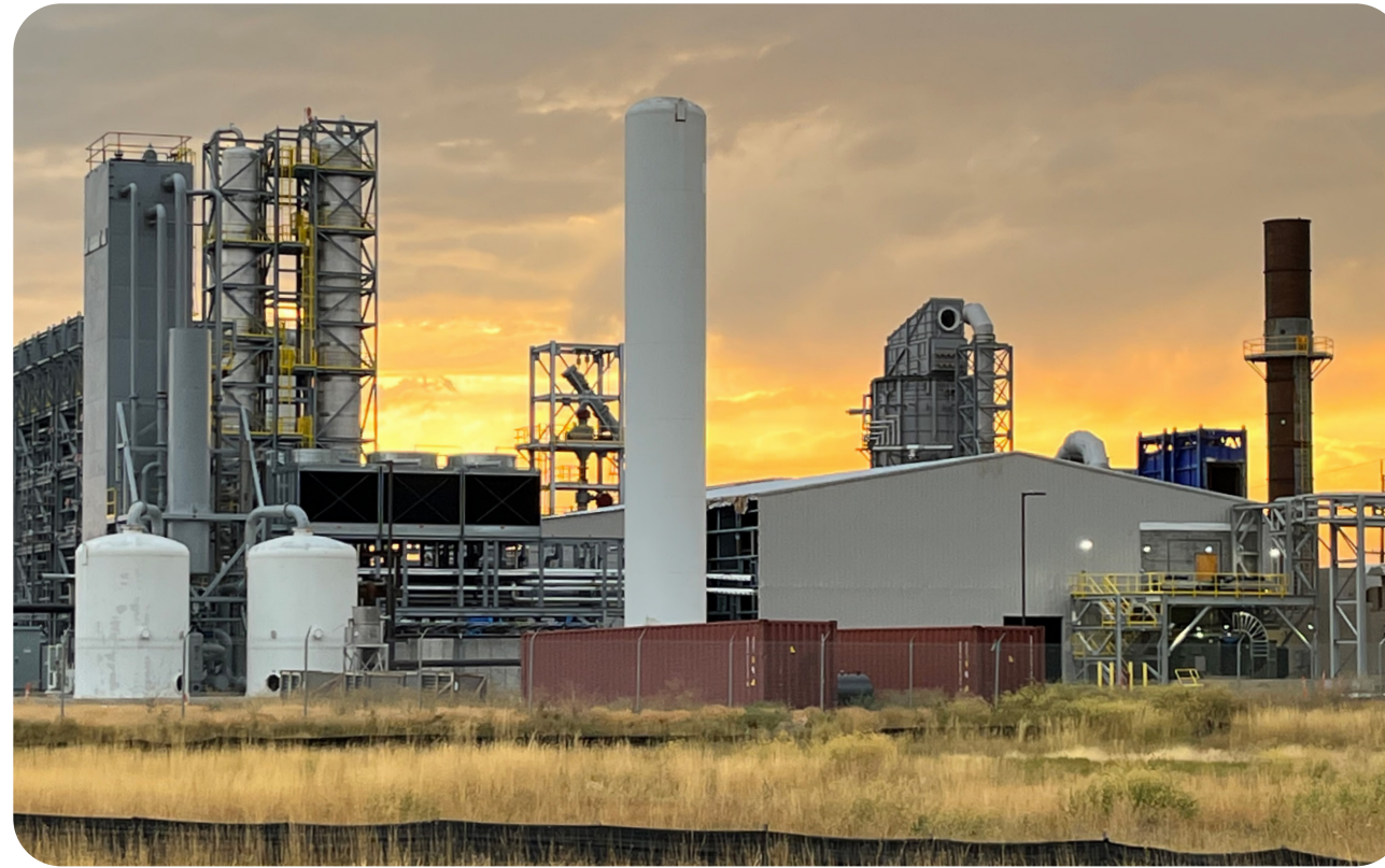
Lakeview RNG Facility
